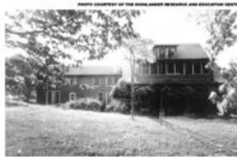
Highlander Folk School Main Building, Monteagle, TN.
