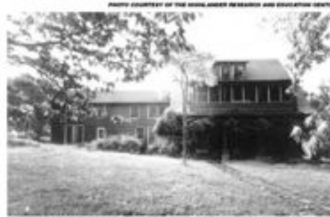
Highlander Folk School Main Building, Monteagle, TN.
