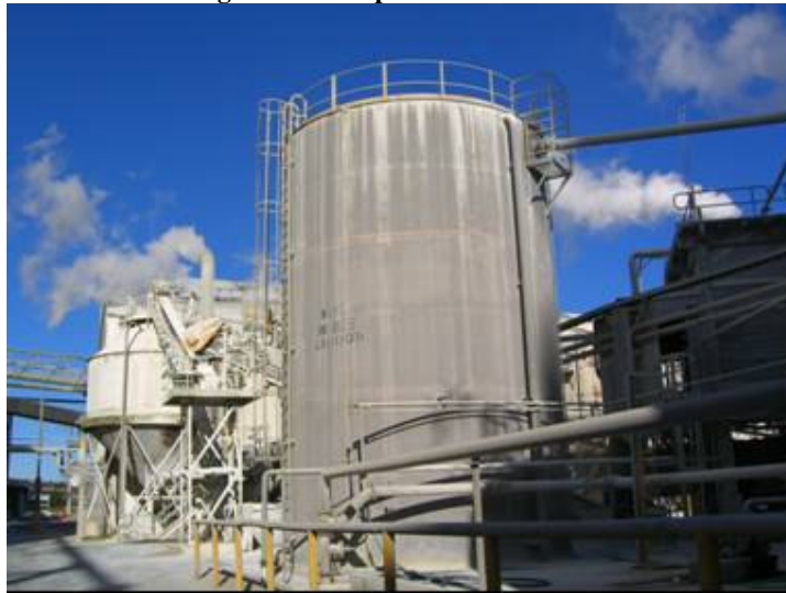
Figure 0-16: White Liquor Tank
